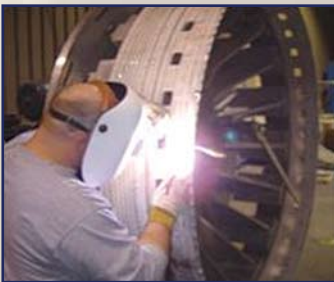
Certified Weld Repairs
